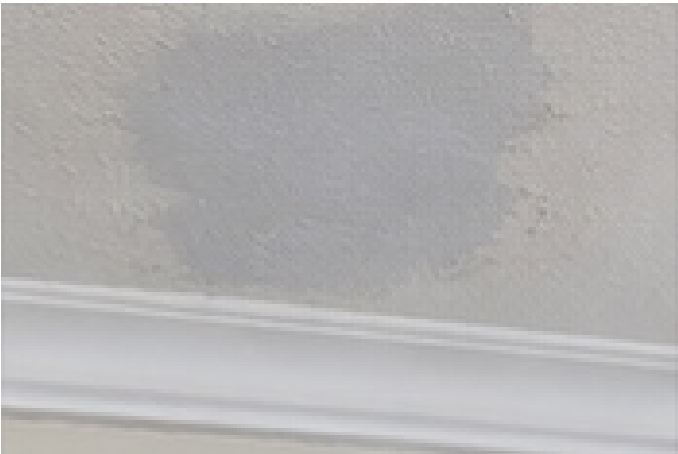
Repair in progress · 2:06 pm
